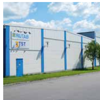
Warehouse - and production facility in Nässjö, Sweden
